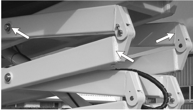
Figure 7.19 - Structural Damage and Welds
